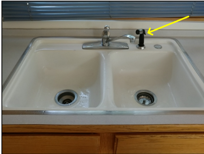
Sprayer is nonfunctional.
