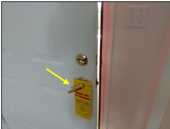
Front door lockset: adjust/replace or repair.
