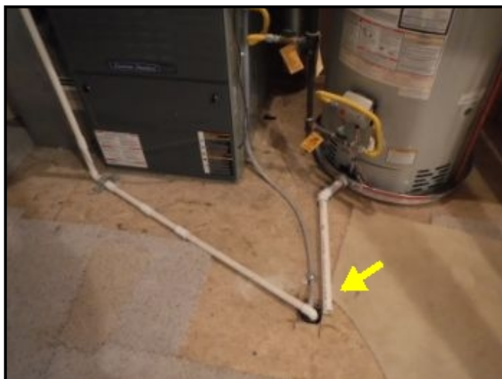
PVC should be directed into ABS drain.
