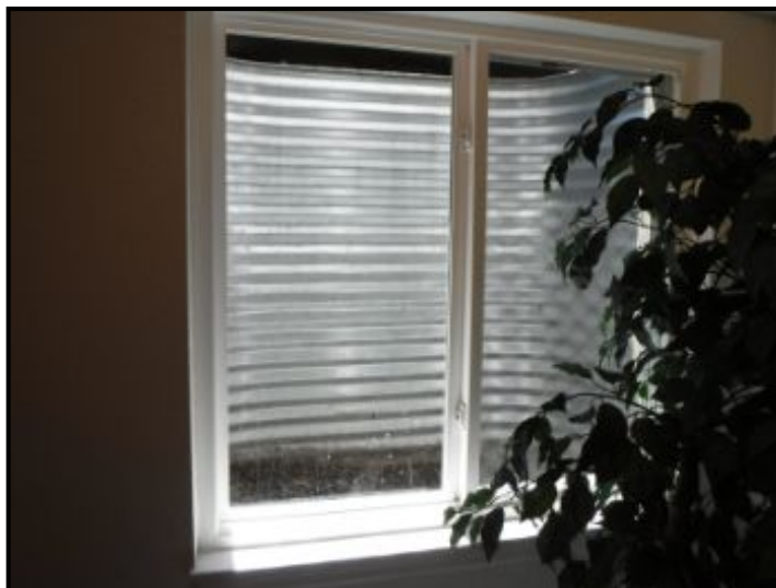
Install ladders as needed in window wells.
