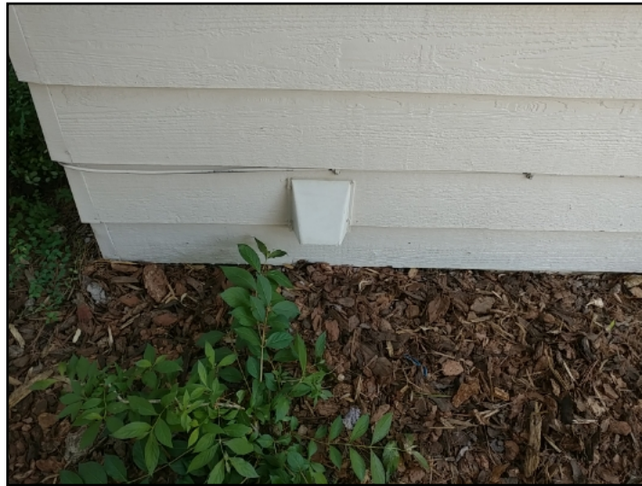
Dryer vent. Functional.
